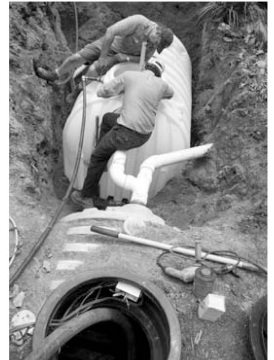
Installation of rainwater-collecting cisterns, 2008.
